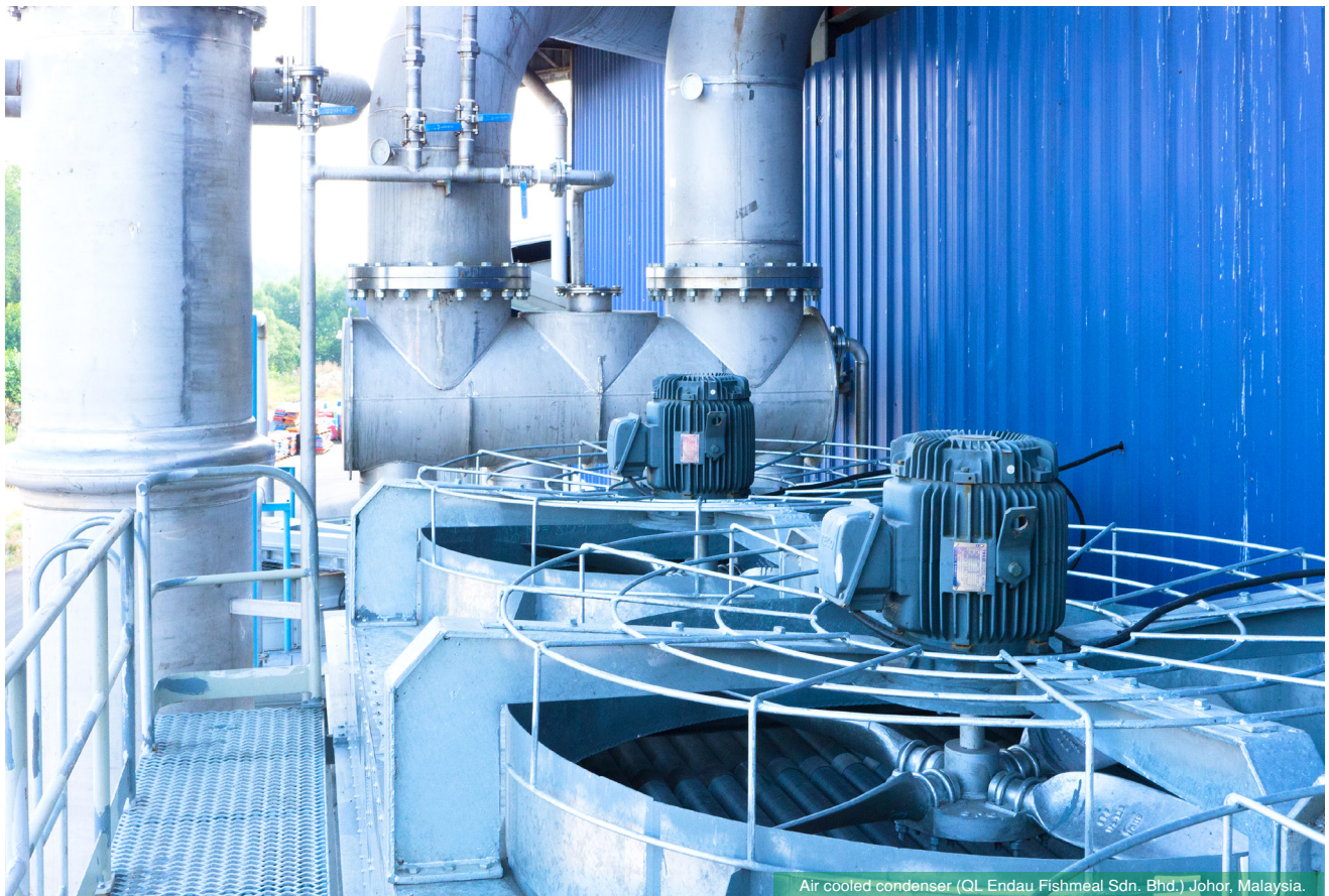
Air cooled condenser (QL Endau Fishmeal Sdn. Bhd.) Johor, Malaysia.
